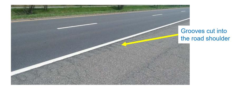
Groove spacing is nearly equal, so noise is very tonal
